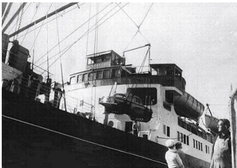
A car being slung onto the Taroona
